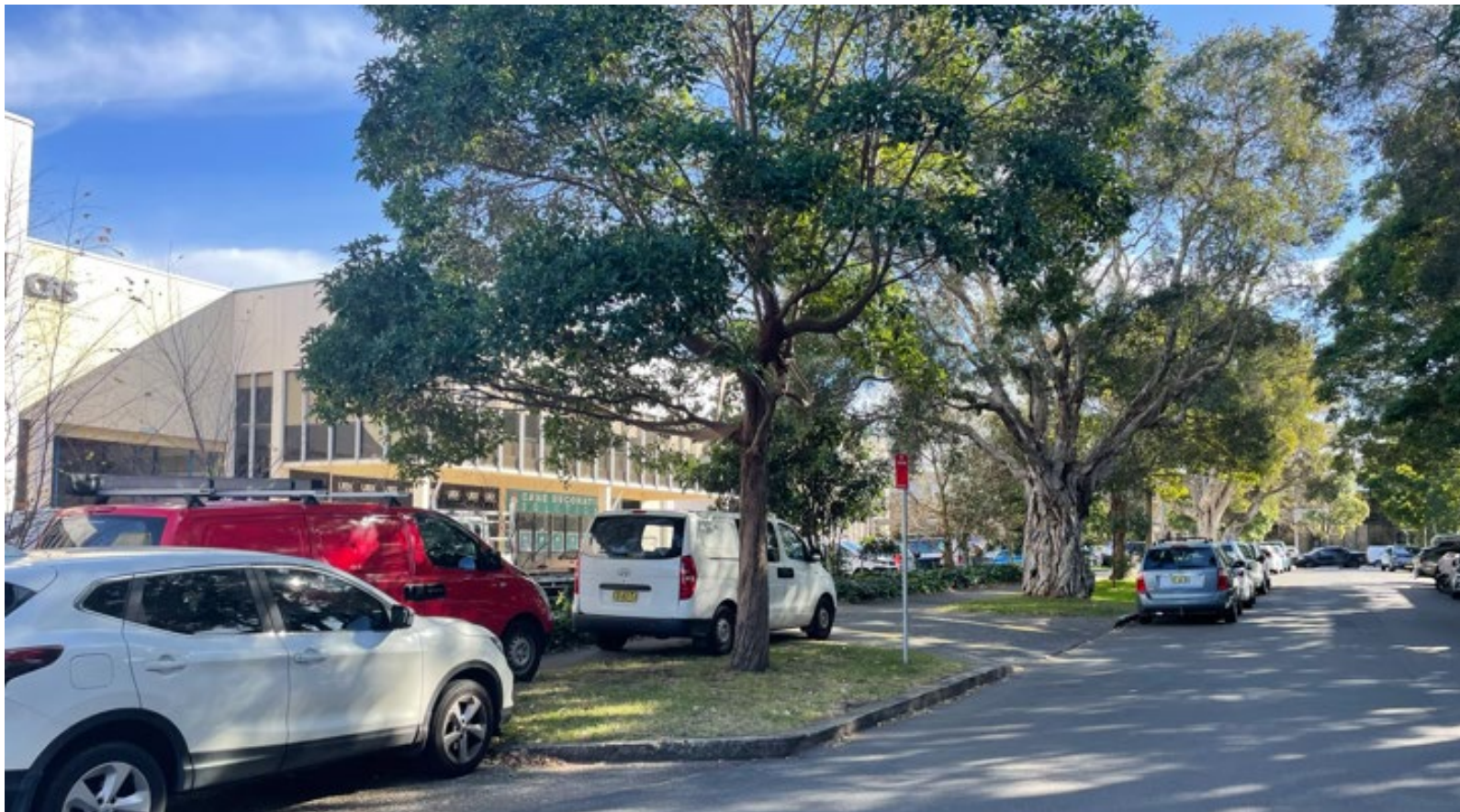
warehouse development opposite the site Stokes Avenue
